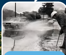
Flooding on Front Street in 1974.
